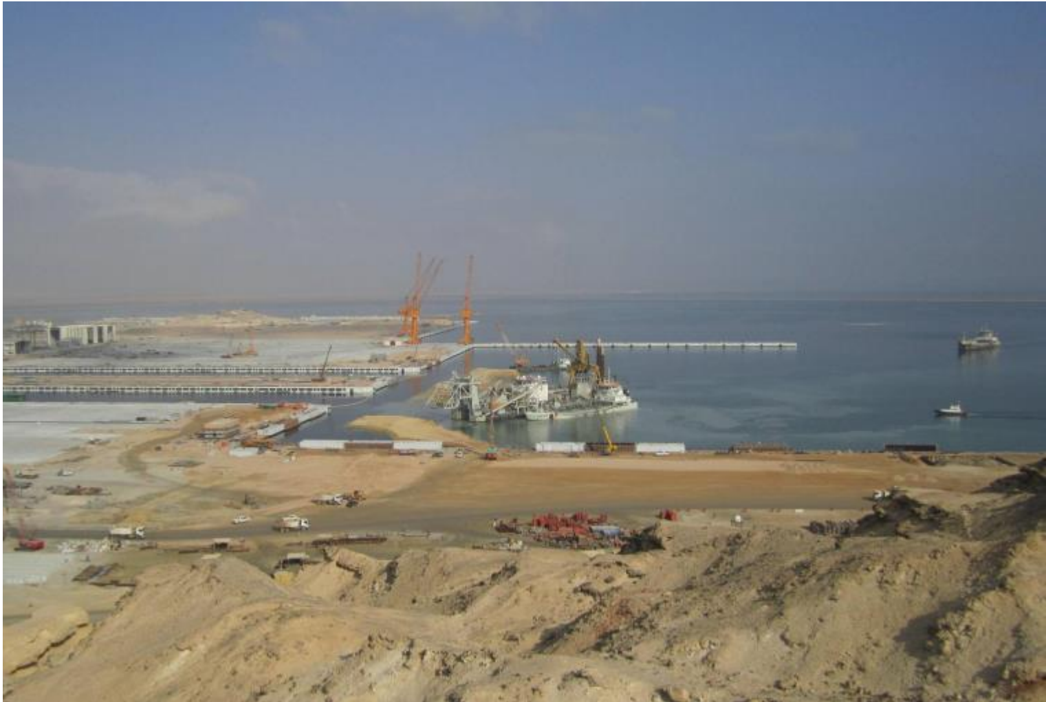
Oman - Construction of New Port Complex in Duqm
